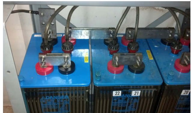
Fig 3. Manifold Vent System
