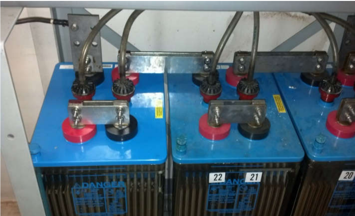
Figure 4. Manifold Vent System
